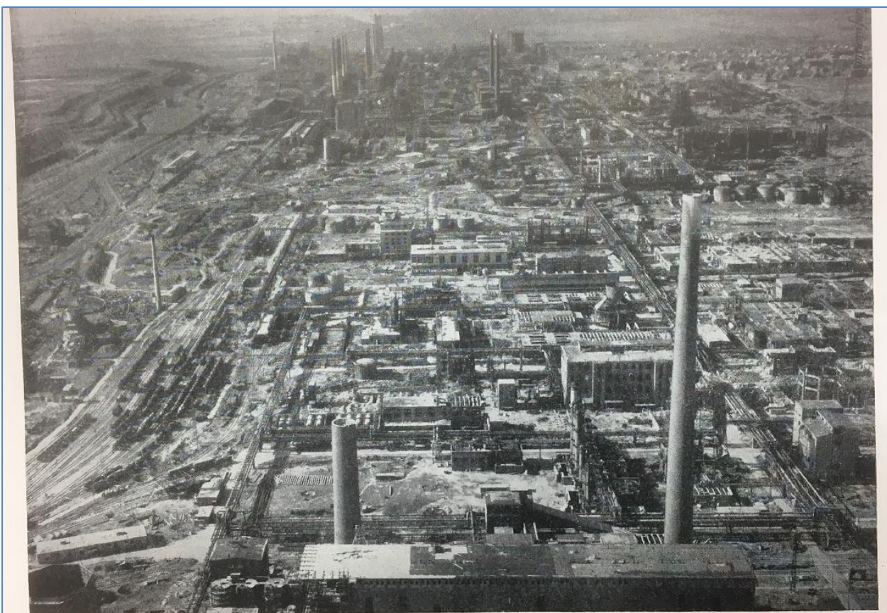
Figure 117. View of Leuna Works, taken by the Eighth Air Force in May, 1945. Fore-ground, the organic products division. Right middle distance, the hydrogenation area. The group of 11 chimneys in the distance marks the older boiler and power plants. To the left of them is the gas production area.
