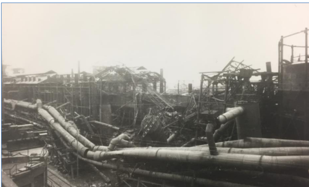
Image 7: Extensive damage to pipe racks in Leuna following air raid.
