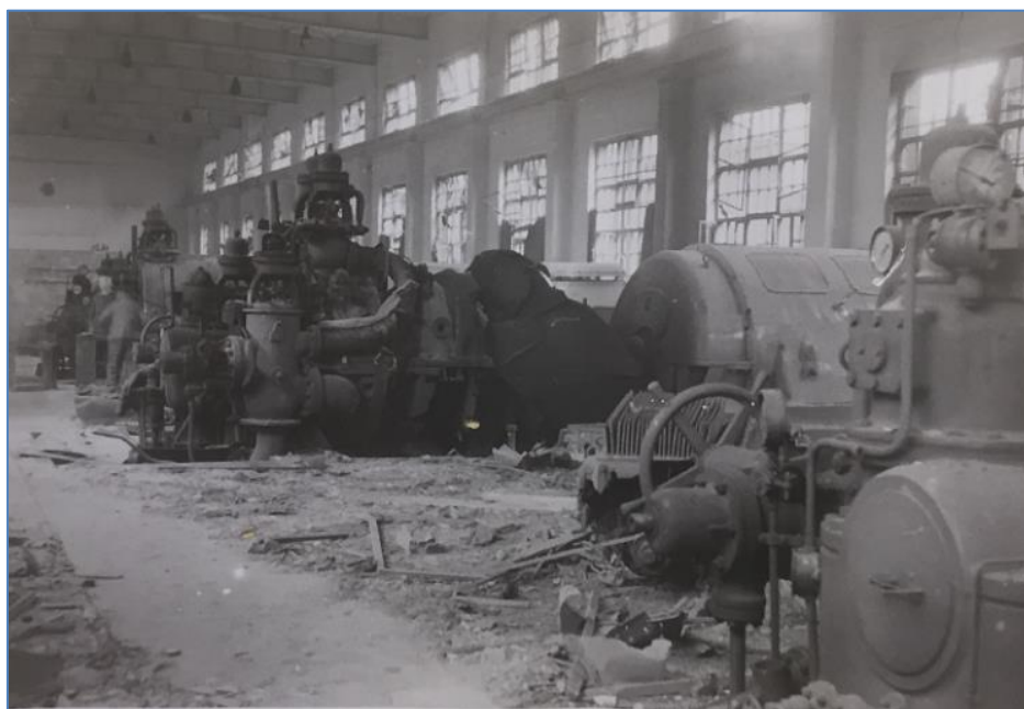
Image 8: Limited damage to buildings and equipment in Leuna following air raid (Building Me 5 13 May 1944). Source: LASA, I 525, No. A 1509
